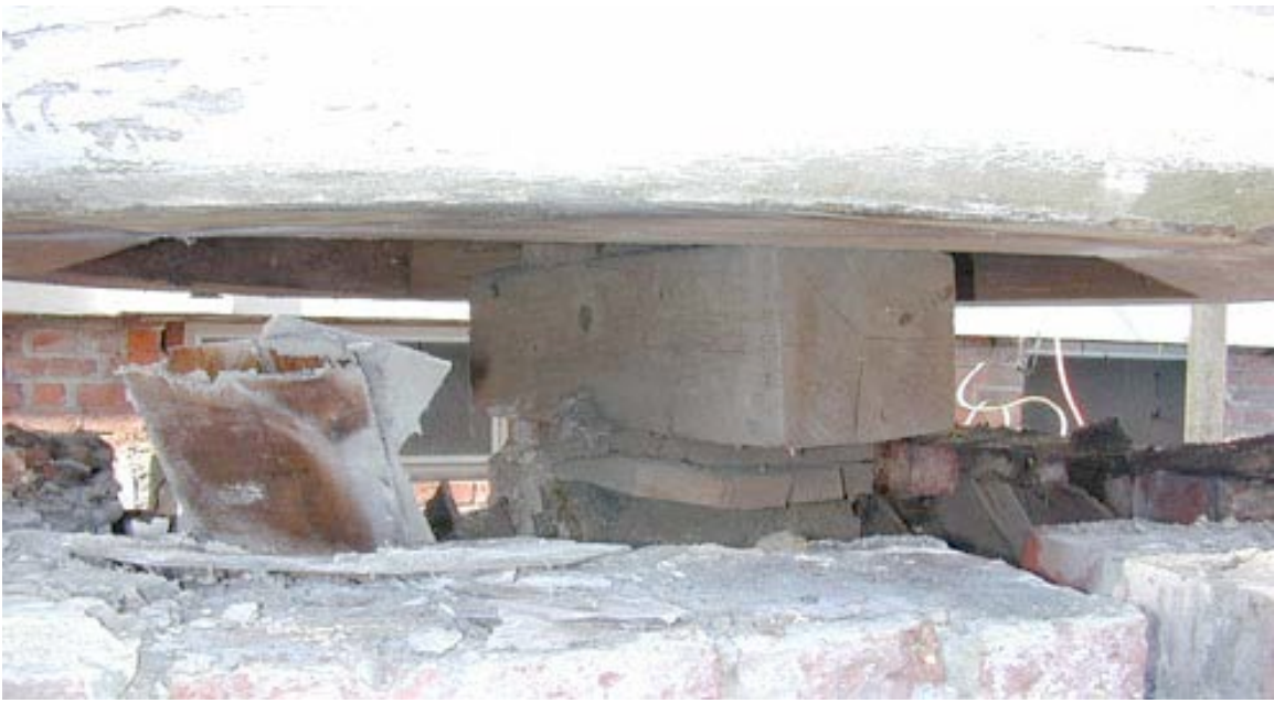
Figure 21: all manner of supports were used over time
