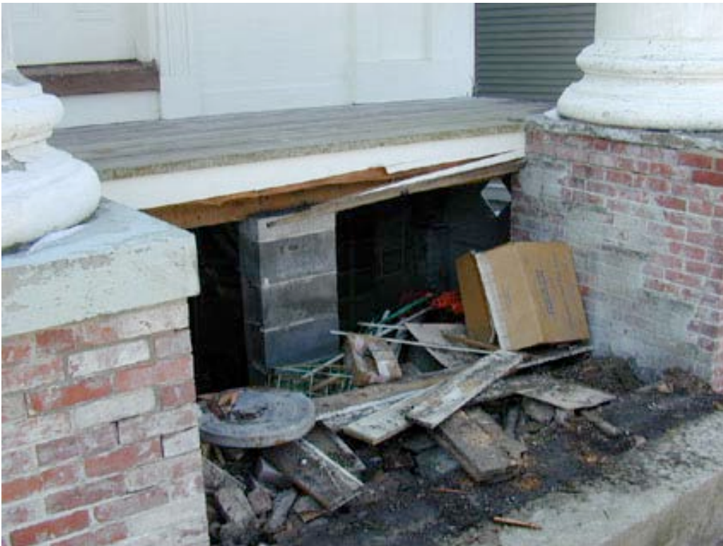
Figure 13 and 14: Steps removed prior to demolition and staging. The bases were made of three different materials: granite for the outer columns, concrete on the right two, and wood on the left.
