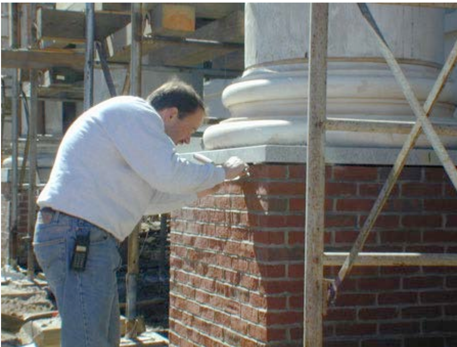
Figure 42: Final mortar is applied beneath granite cap
