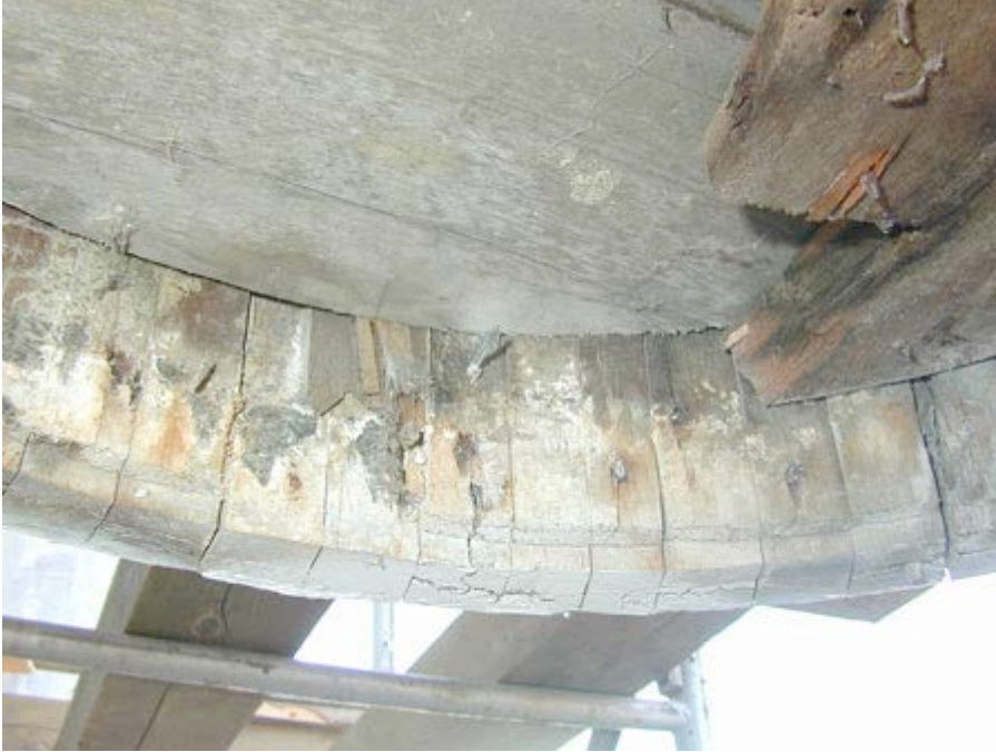
Figure 23: Removal of the bases allowed for inspection of the bottoms of the columns. Here the wood is largely intact. Note that rabbeting was used to secure column to base
