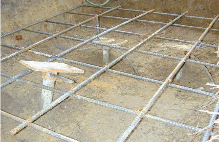
Figure 27: 3 anchor caps and rebar are welded together before footing is poured.
