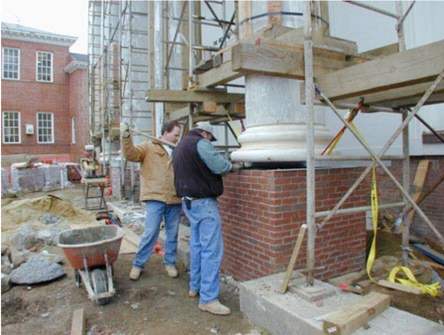
Figure 41: Mortar bed is applied before granite slab is repositioned.
