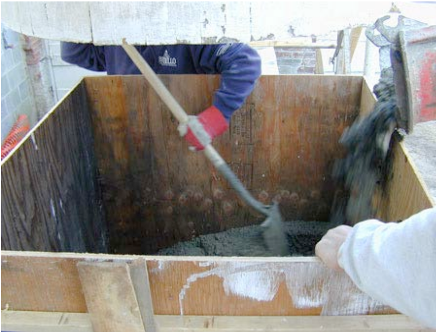
Figure 30 and Figure 31: Forms are filled with concrete mix
