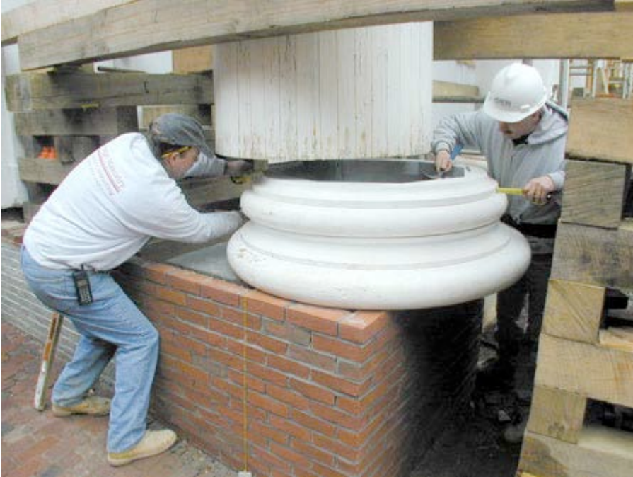
Figure 37: The new mahogany base is fitted into place but will remain suspended until the granite cap for the pedestal is finally positioned.
