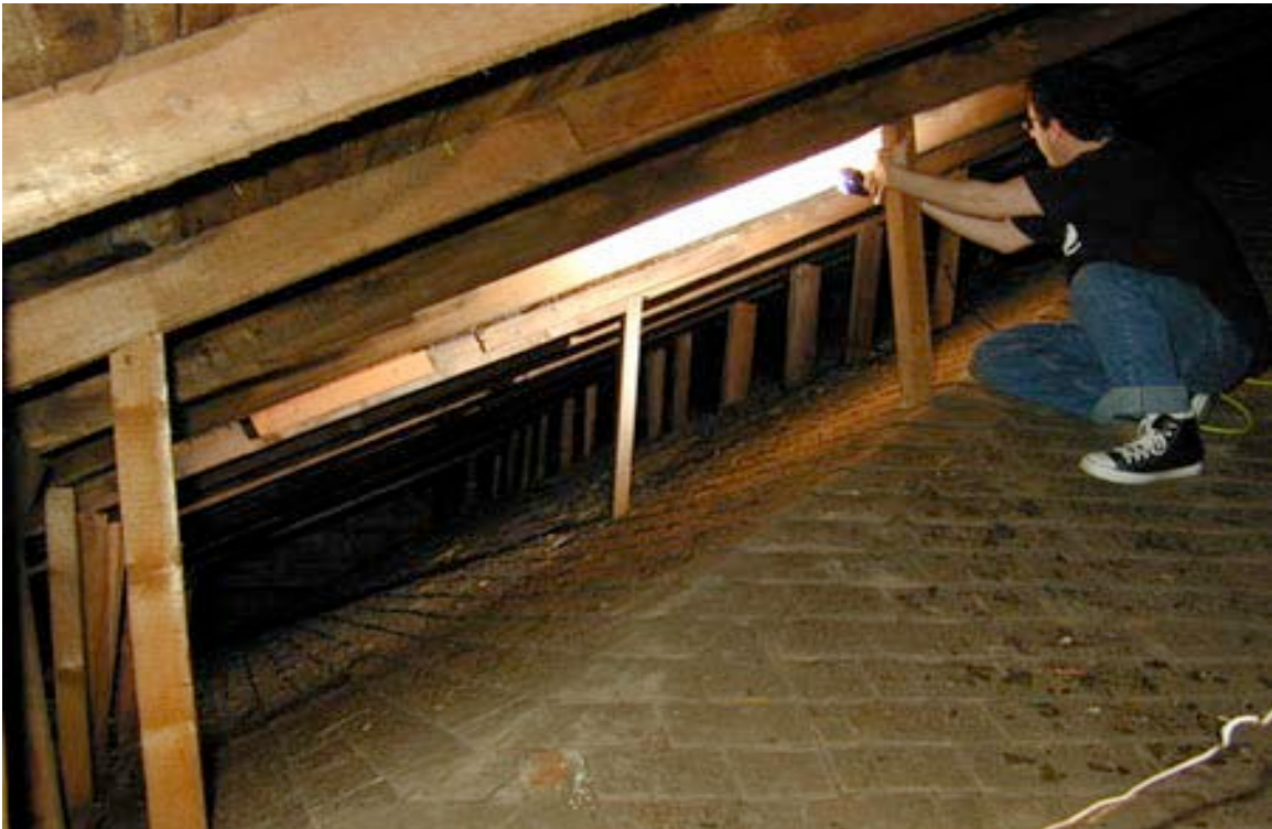
Figure 1: Standing on hipped roof with gable roof above
