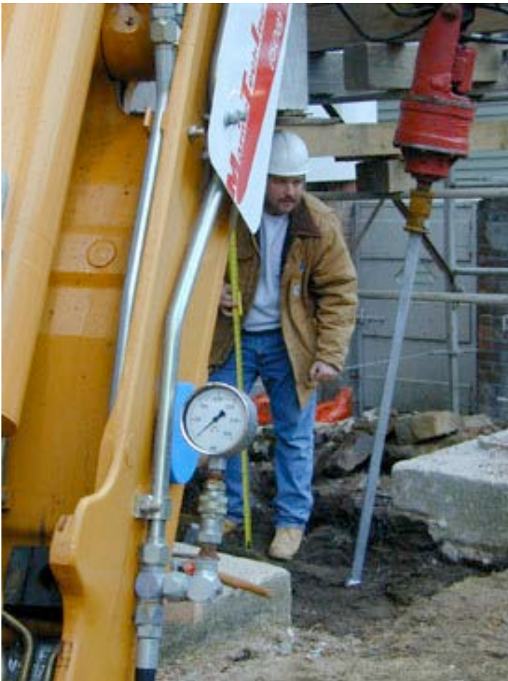
Figure 25: The first helical support is positioned
