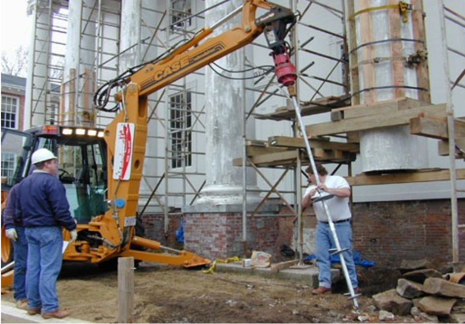
Figure 25: The first helical support is positioned
