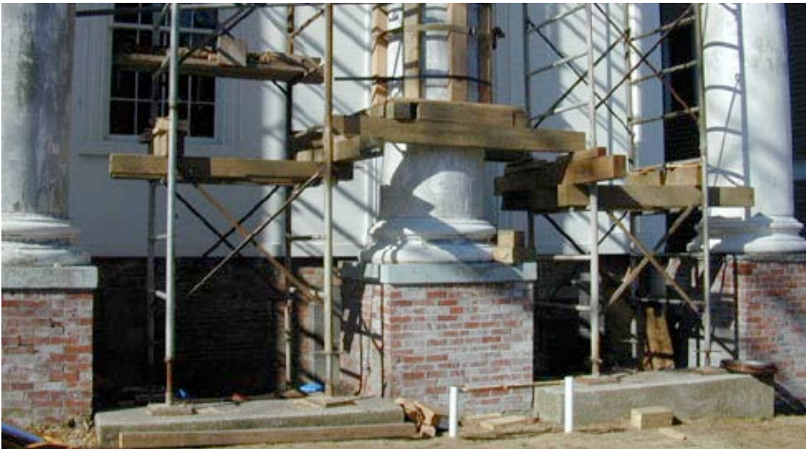
Figure 23: Removal of the bases allowed for inspection of the bottoms of the columns. Here the wood is largely intact. Note that rabbeting was used to secure column to base
