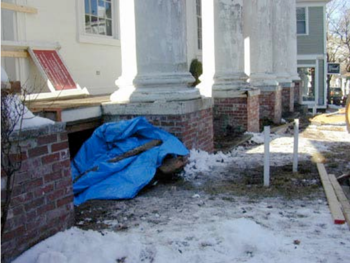
Figure 13 and 14: Steps removed prior to demolition and staging. The bases were made of three different materials: granite for the outer columns, concrete on the right two, and wood on the left.
