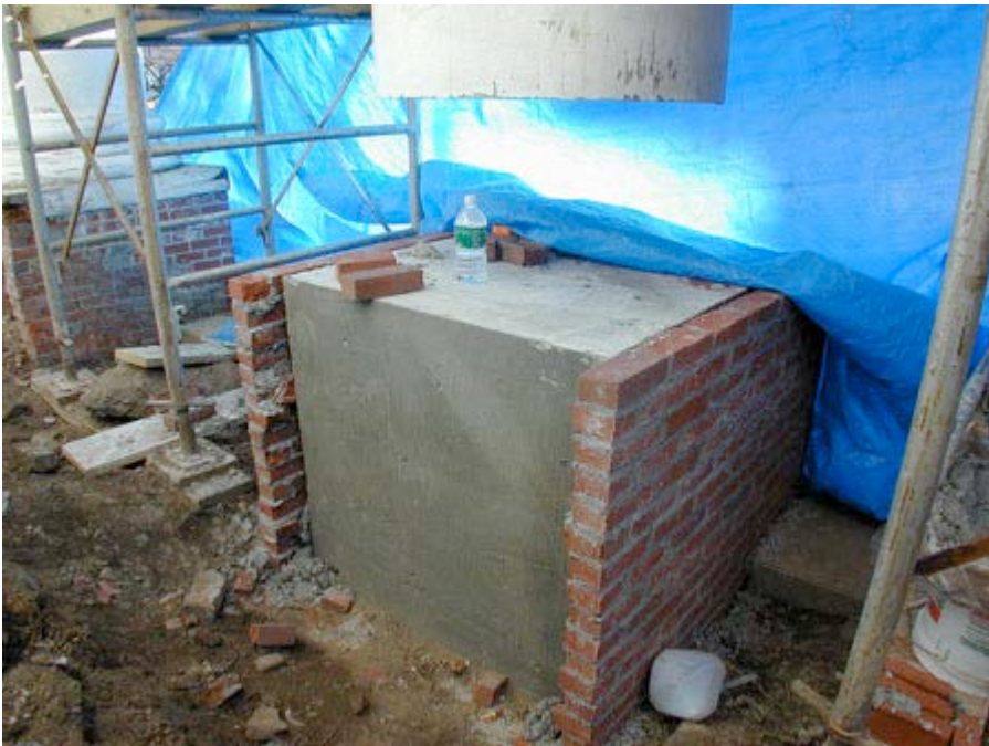
Figure 36: The back of one of the reconstructed pedestals prior to the acid wash
