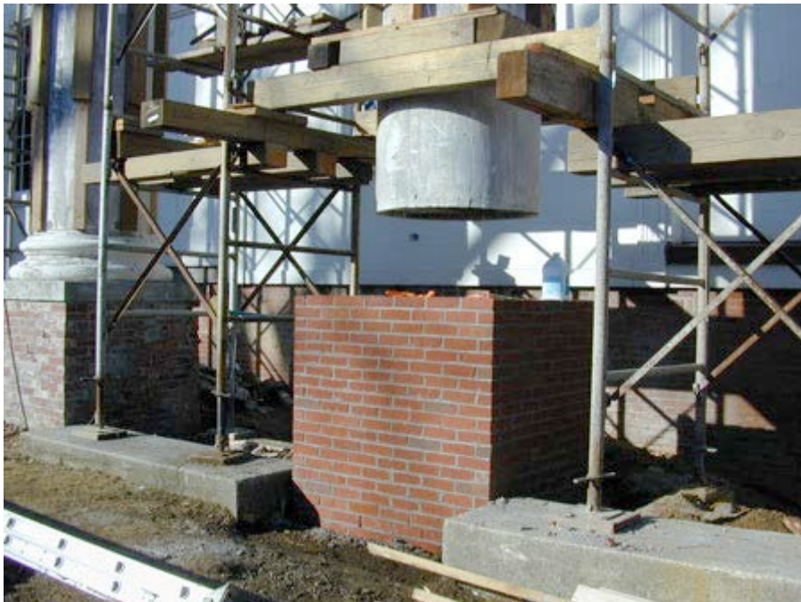
Figure 33 and 34: Mortar samples were made up by the mason for LPC approval based on the mortar analysis report provided by Jablonski-Berkowitz Conservation in New York. While the color and texture were matched, the hardness was made to be compatible with the new brick selected to face the pedestals.
