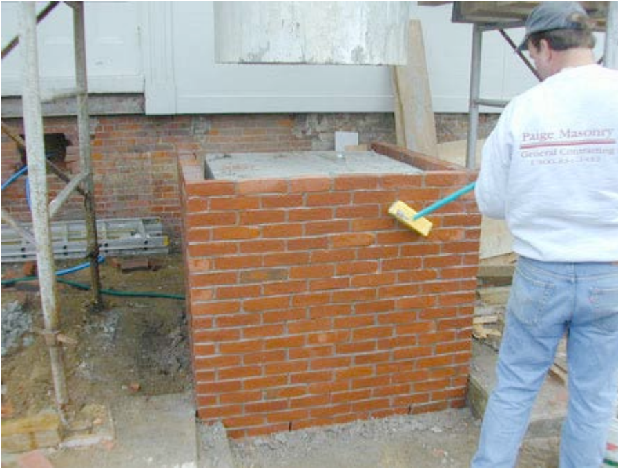
Figure 35: An acid wash over the brick removes final debris
