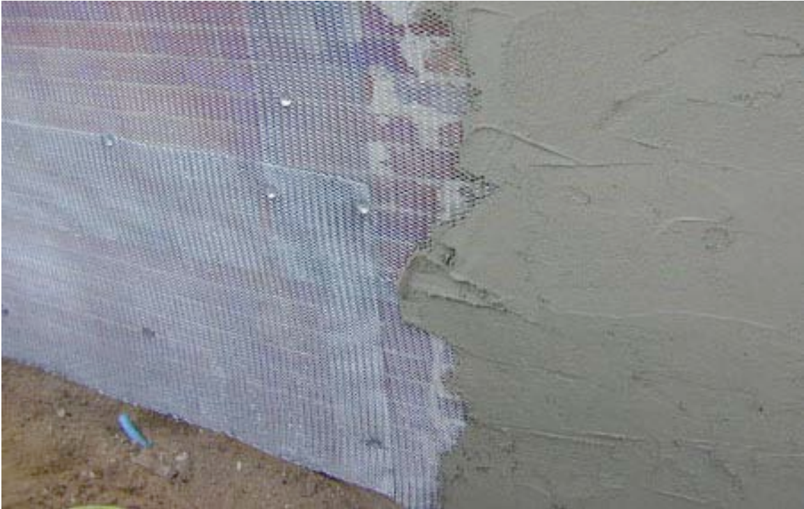
Figure 43: A skim coat of parging is applied to front façade foundation
