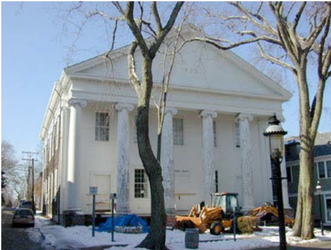
Figure 12: Weather conditions allowed work to proceed in late January, 2000
