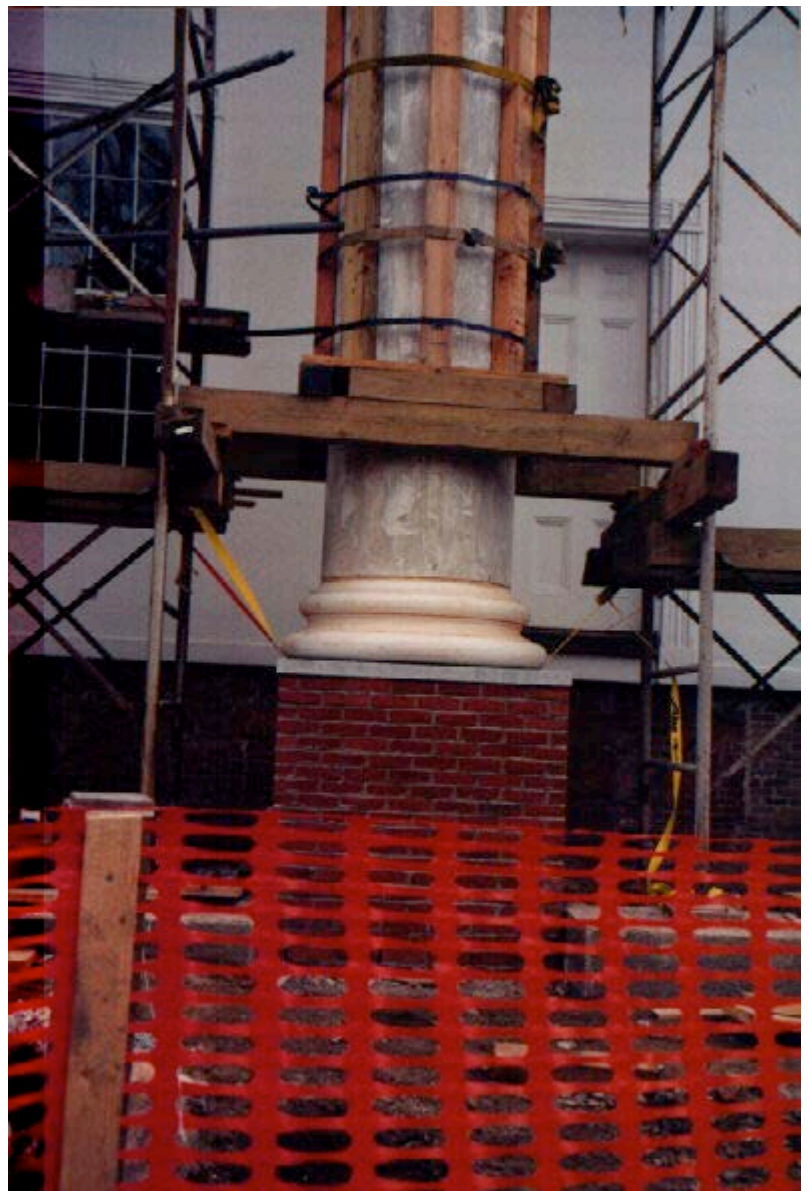
Figure 40: The column remains braced so no movement or shifting can occur
